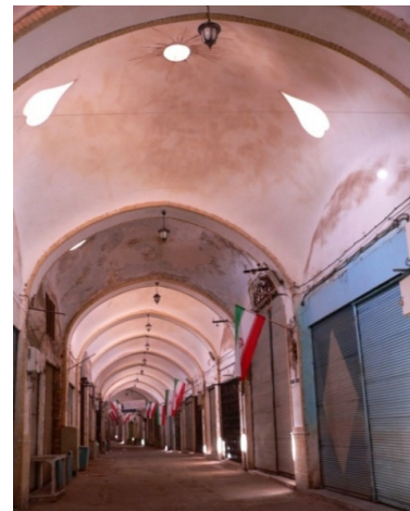
The space in front of Haj Asgar bathroom
