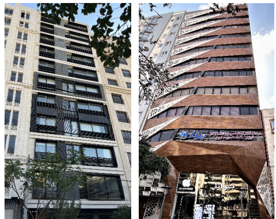
Facade with two-dimensional form and wood and metal materials
