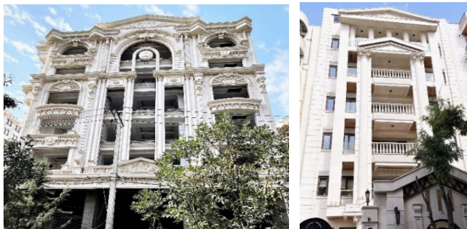
Facade with three-dimensional form and stone materials
