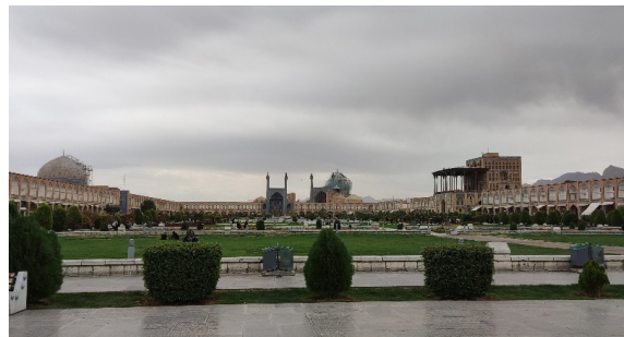
Figure 10 : View of floor, wall and roof of Naqsh Jahan square
