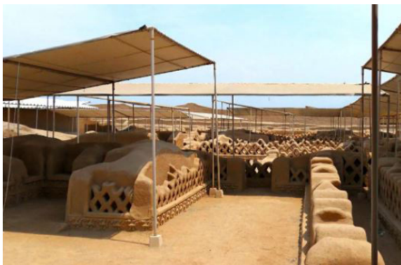
Fig. 12: Roof cover to protect rainwater. Photo by R. Orazi.
