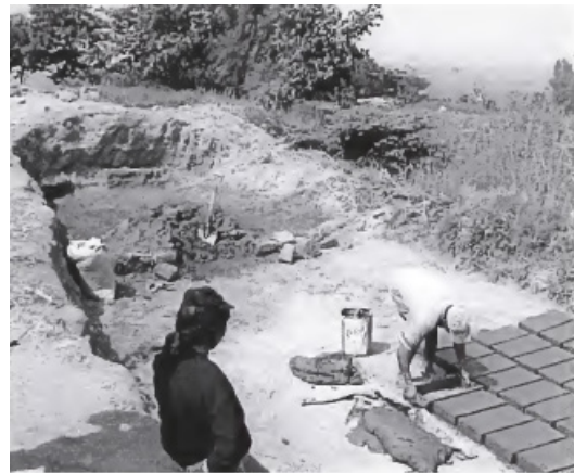
Fig. 13: How to make and mold adobes and dry them in the sun, Source: (L.Smailes, 2020, p. 36)
