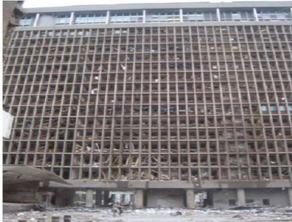
Figure 2: Failure of windows in Terrorist attack in Oslo, 2011 (Larcher et al., 2016)
