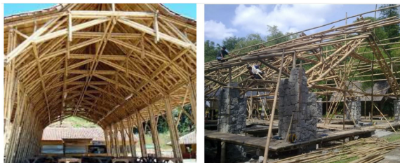
Figure 9: Construction of bamboo truss (Hildayanti and Wasilah, 2023).
