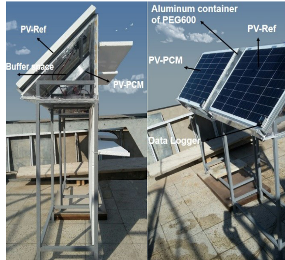
Figure 3: Installation of reference PV and PV PCM systems
