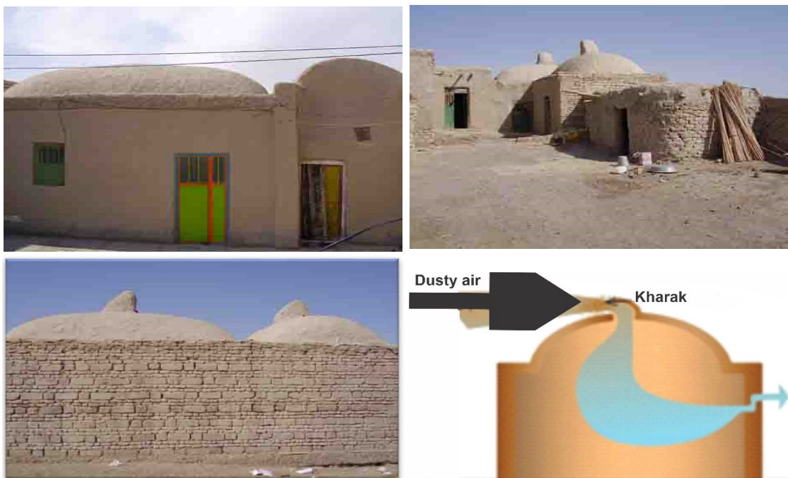
Figure.2: Separation of animal and human spaces in Sistan and the combination of dome roofs and windbreaks in Sistan
